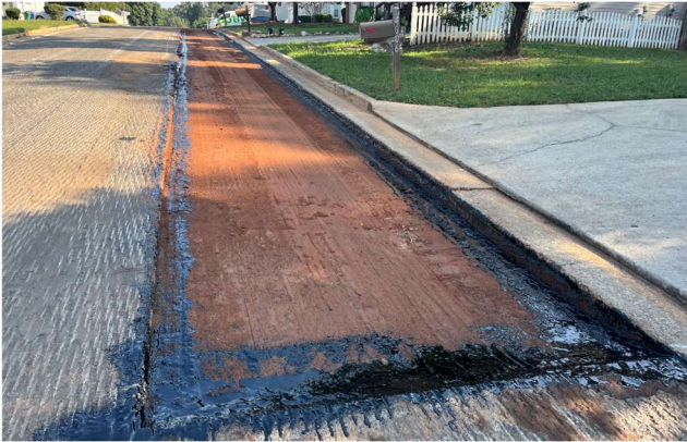
Roads with most the base and subbase missing.
